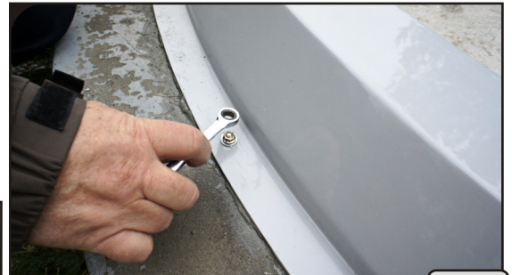
Tightening Hilti anchor
