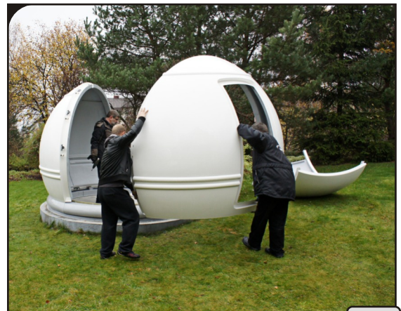
Assembling the dome on the concrete slab in the garden
