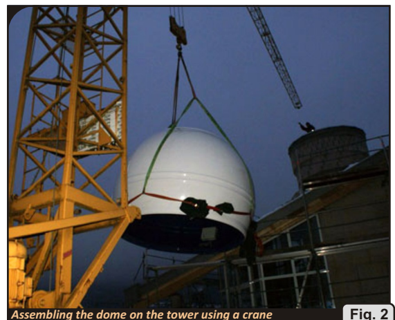
Assembling the dome on the tower using a crane
