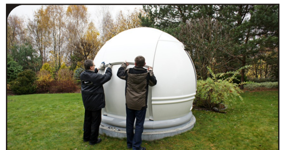
Putting the shutter on the dome
