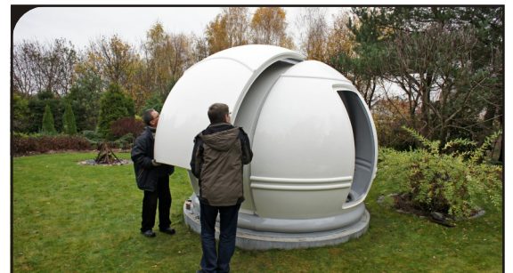
Putting the shutter on the dome
